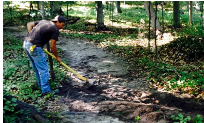
Water boards were added along the trail at Whaleback Natural Area to prevent erosion on steep slopes. Note the tree roots exposed where volunteer Marc Vargas creates the water diversion trench.
