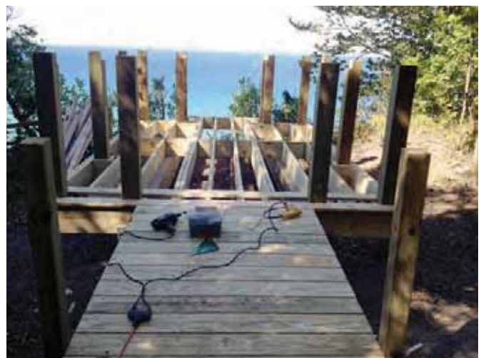
Clay Cliffs observation platform in progress
